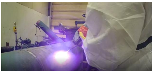
Manual operation in a confined area: Asbestos fibre dispersion: 0 f/l
