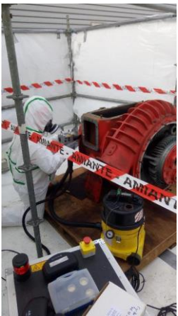
Manual operation in a lightly confined area. Asbestos fibre dispersion: < 10 f/l
