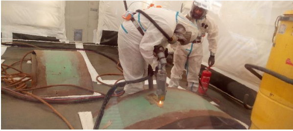
Manual operation in a confined area: Asbestos fibre dispersion: 3 f/l
