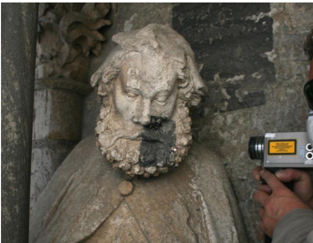
Removing the dirt of the millennia without damaging the material (Ulm Cathedral)
