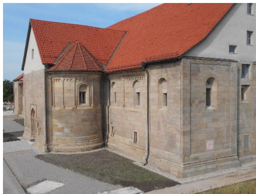
Sandstone facade of St. Peter's Church in Erfurt after laser treatment
