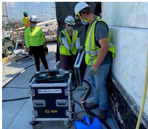
Portable CL 100 in a robust housing with easy-to-use processing optics
