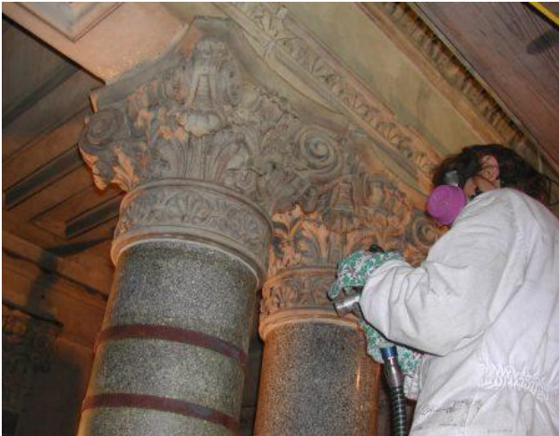
The laser beam reaches even into fine recesses
