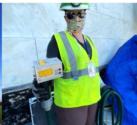
cleanLASER in action at the Jefferson Memorial in Washington: Sustainable removal of the dark biofilm on the historic marble with the CL 100
