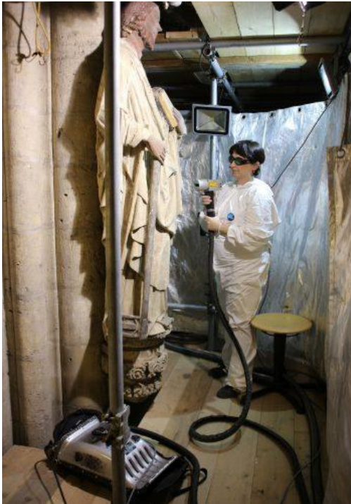
The backpack laser in action - it can be used as a backpack or like a "cleaning vacuum cleaner" (Photo: DBU)
